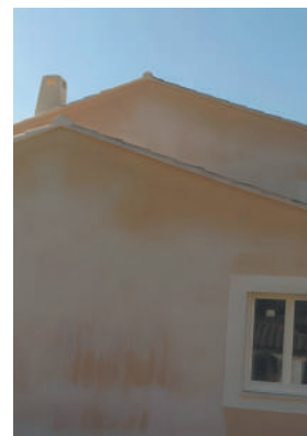
Efflorescence
